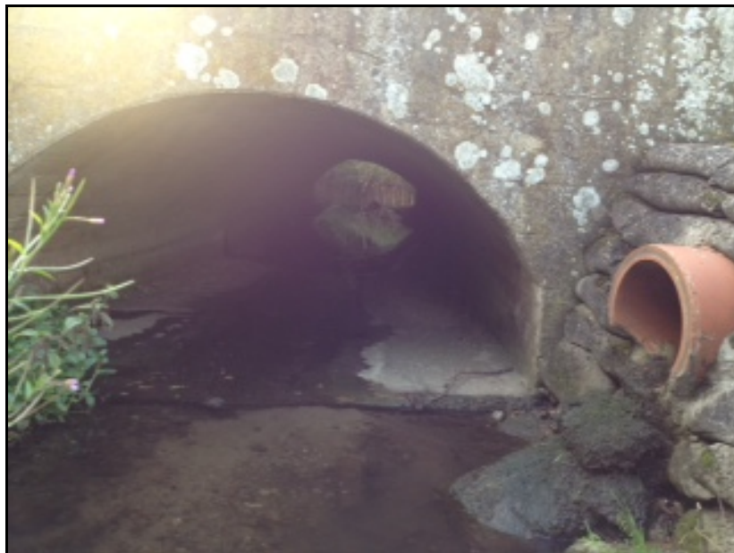
Figure 20: View of concrete bridge under The Street looking downstream (Source: [REDACTED] 3/8/2012)
