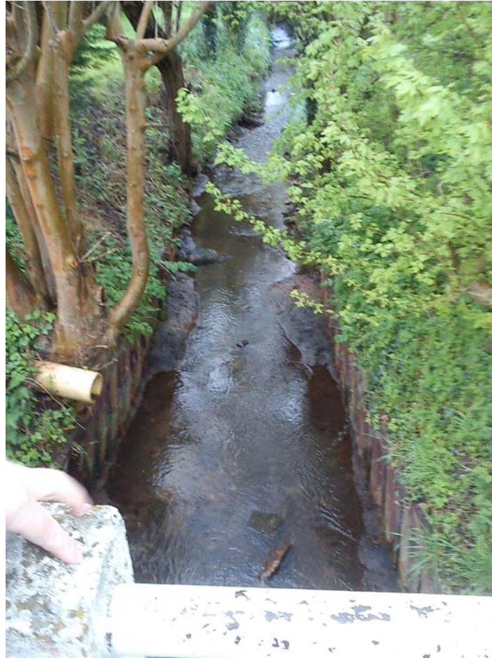
Figure 2: View of watercourse looking downstream from bridge (at The Street) (Source: Evans Rivers and Coastal taken 3/5/2012)
